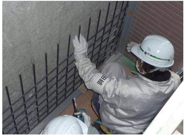
組立鉄筋取付
